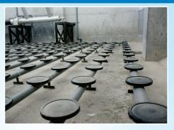
Fine pore flexible membrane diffusers provide operational flexibility with maximum oxygen transfer efficiency for aeration tank.
